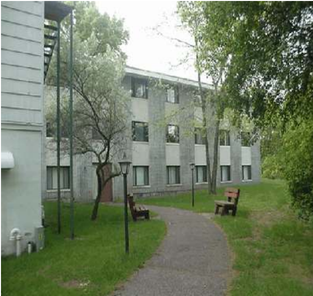
SOUTH HALL Girls' Dormitory
